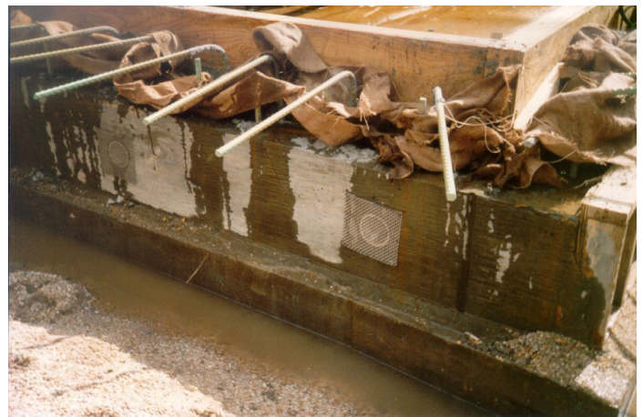
Weep holes with screens to control seepage.
