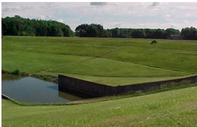
Properly maintained embankment.
