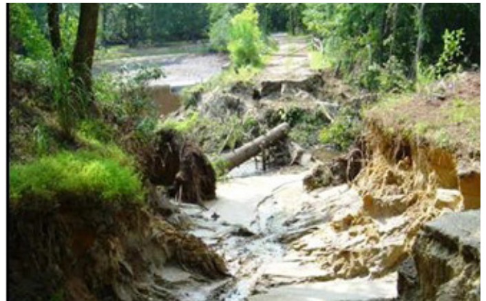
Above: Seepage that developed where the root ball of a tree pulled out of the ground near the downstream toe of the dam.
