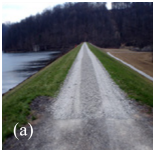
(a) Crest with a good cover that will reduce the effects of vehicular traffic.
