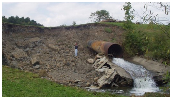
Above: Corroded corrugated-metal outlet pipe removed from a dam that had developed large sinkhole.
