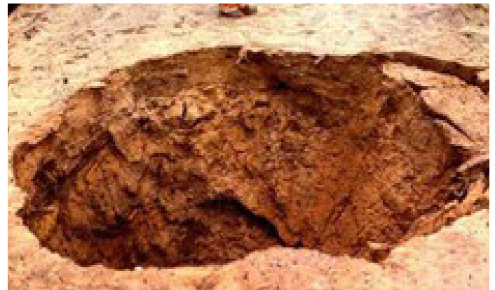
Above: Sinkhole on the crest of an earth dam. The reservoir was lowered and a cavity was found under the sinkhole.
