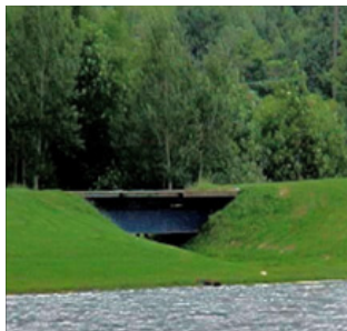
This bridge blocks much of the spillway, reducing its ability to convey water.
