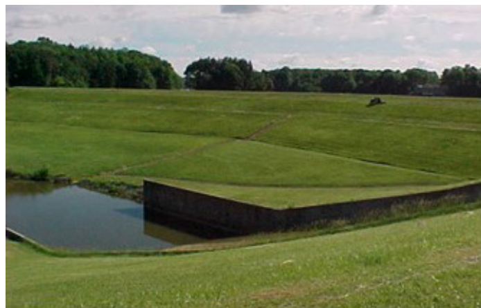
Properly maintained embankment.
