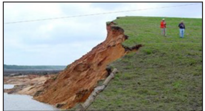
Failure at a dam caused by internal erosion of the soil abutment.
