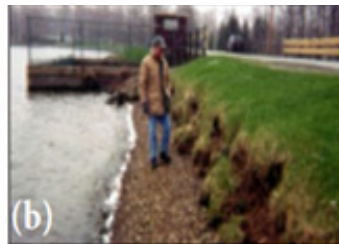
(a) Collapsed muskrat burrows increase shoreline erosion and sloughing. (b) This shoreline has eroded due to lack of proper erosion protection leading to sloughing and cracking of the slope.
