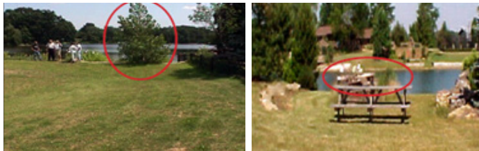
Left: A tree is obstructing this spillway. Right: Notice the landscaping directly behind the table. Obstructions in the spillway reduce the capacity to convey water. They also can collect debris, further diminishing the capacity of the spillway.
